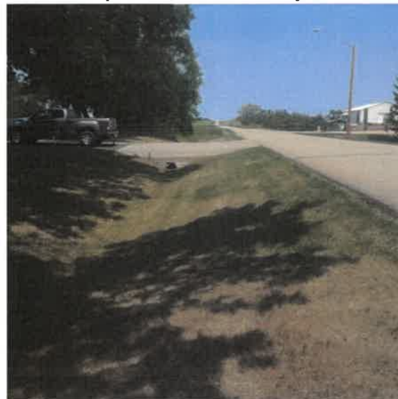
Example – Urban Roadway Ditch
